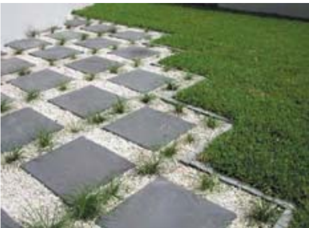
Figure 25 Pavers laid apart for water permeability
